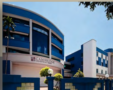
511 & 513 Yishun Industrial Park
