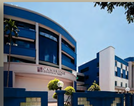
511 & 513 Yishun Industrial Park
