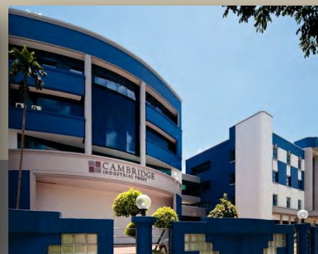
511 & 513 Yishun Industrial Park
