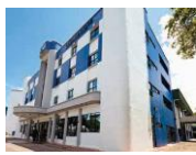
511/513 Yishun Industrial Park A
