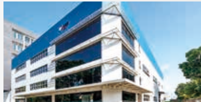
14 60 Tuas South Street 1
