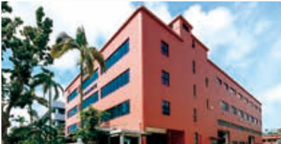
10 31 Changi South Avenue 2
