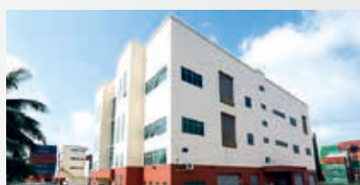
5 79 Tuas South Street 5
