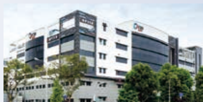
8 30 Marsiling Industrial Estate Road 8
