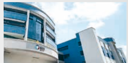
33 511 &amp; 513 Yishun Industrial Park A
