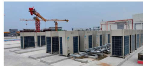
M&E enhancements in progress
