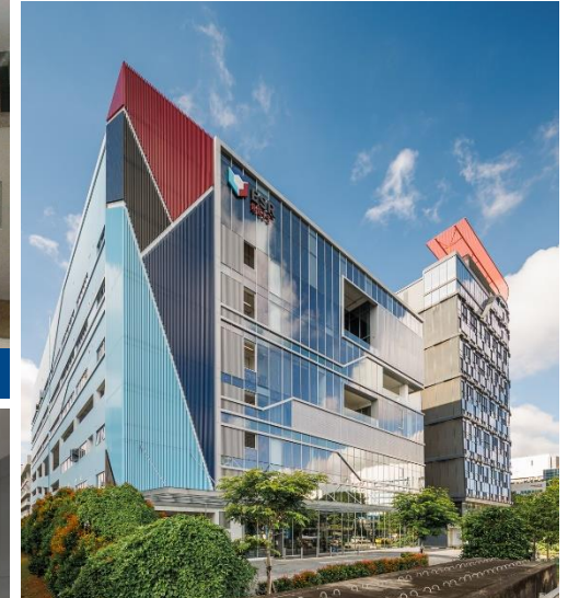
Building façade underwent a major facelift to achieve a modern look
