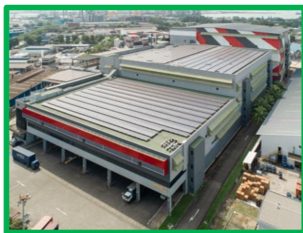
Solar panels installed on the roof of 3 Pioneer Sector 3
