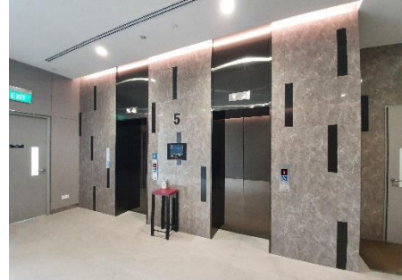
Refurbished passenger lift lobbies
