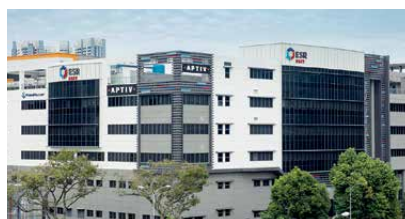
8 30 Marsiling Industrial Estate Road 8
