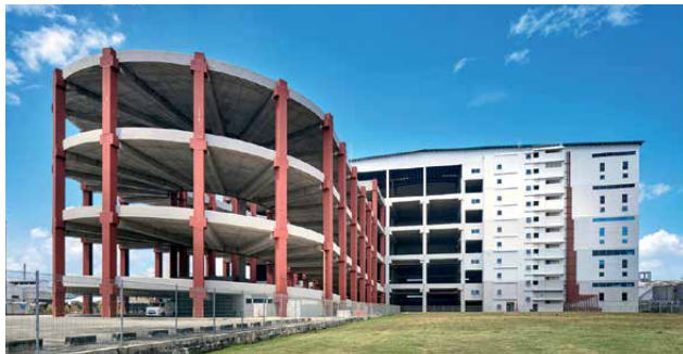
46A Tanjong Penjuru | Logistics & Warehouse
