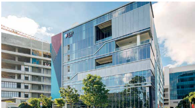
AEI works completed in 4Q 2021
