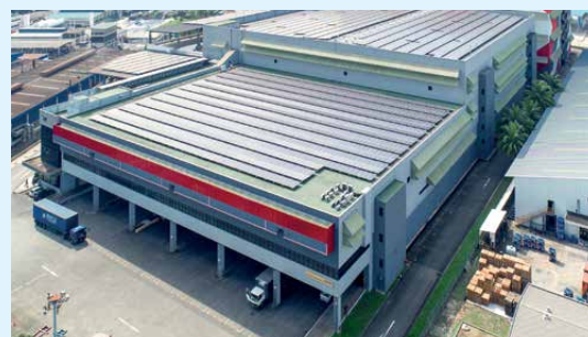
Solar panels installed at 3 Pioneer Sector 3
