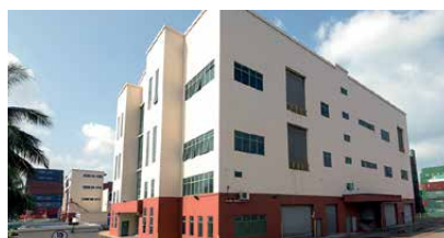
5 79 Tuas South Street 5
