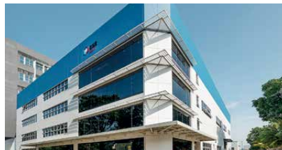
14 60 Tuas South Street 1
