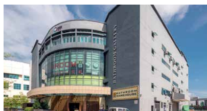
2 25 Changi South Avenue 2
