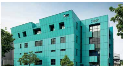
31 45 Changi South Avenue 2
