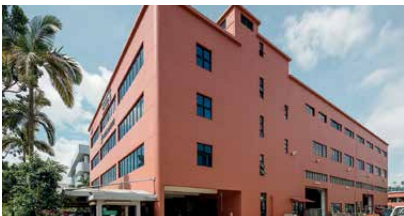
10 31 Changi South Avenue 2
