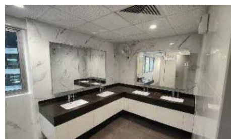
Common toilets after AEI
