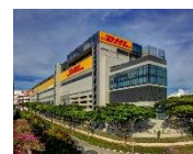
DHL Supply Chain Advanced Regional Centre
